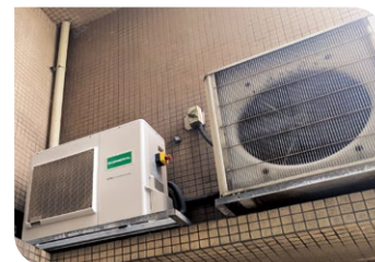
Replaced with new split-type air-conditioning unit
